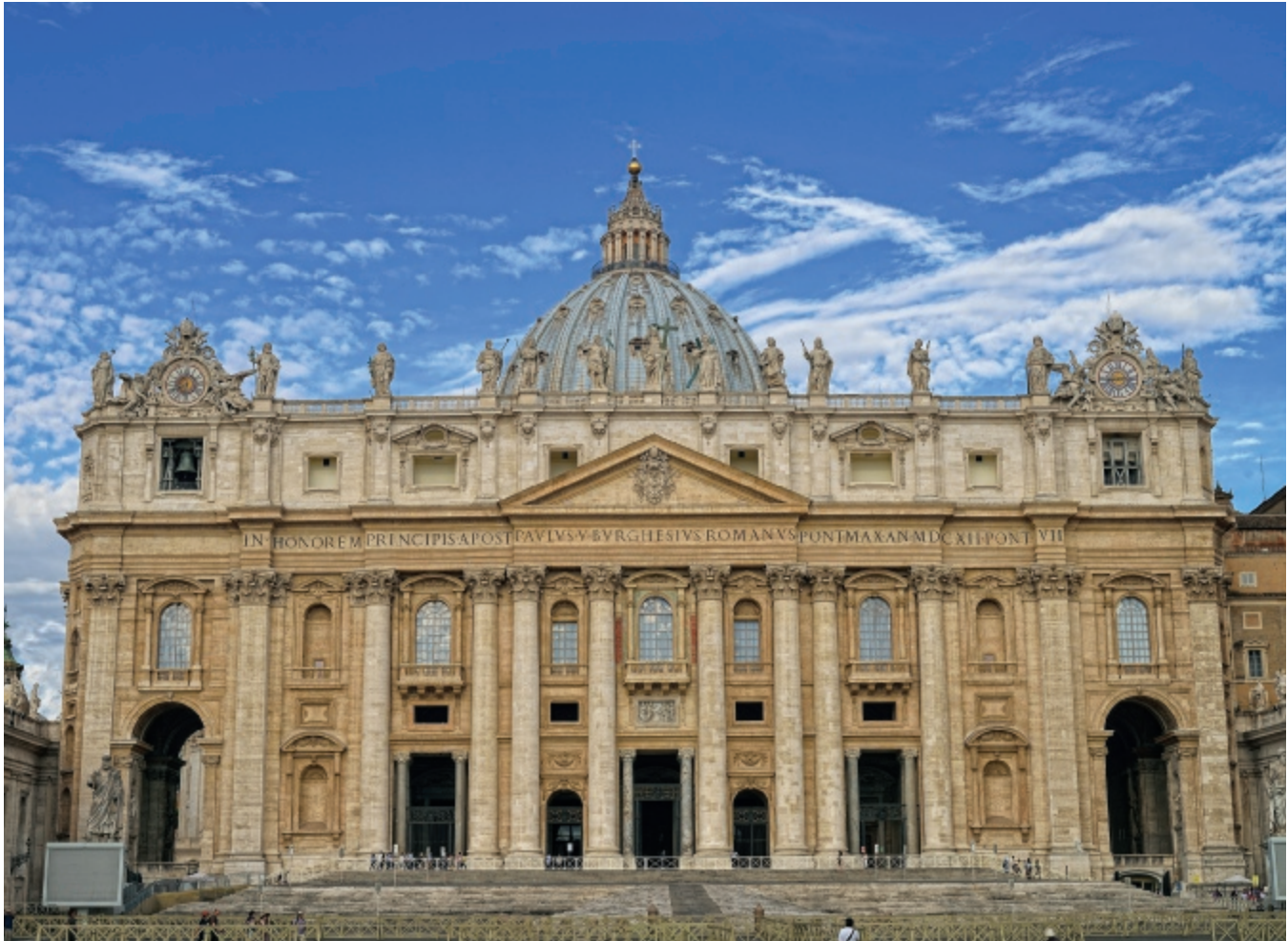
Fig. 21.2 Carlo Maderno, facade of St. Peter's Basilica, Vatican, Rome, 1607–15. Originally the end bays of the facade had bell towers, but because St. Peter's stood on marshy ground, with underground springs, the towers cracked, and they had to be demolished.
